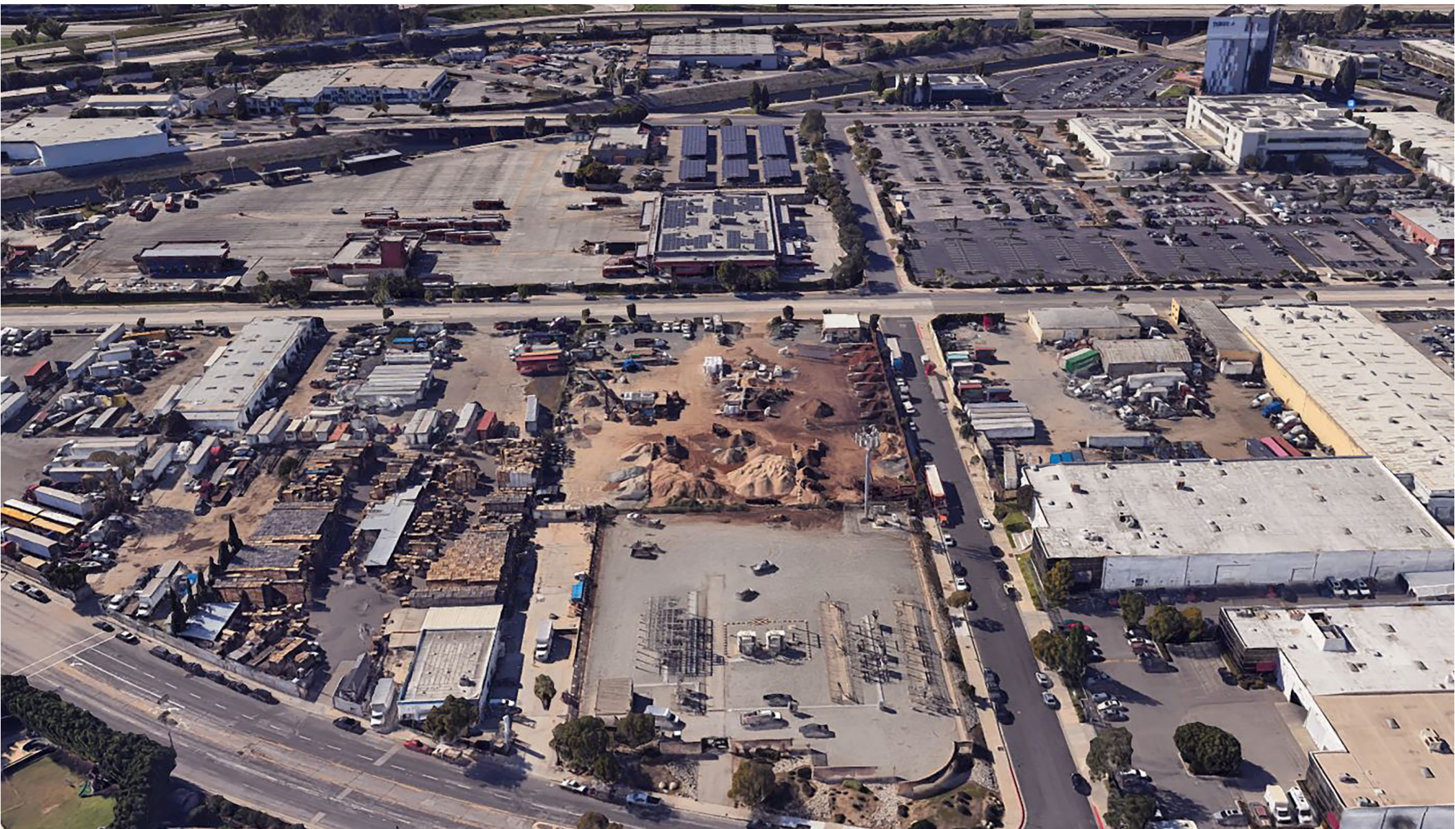
Aerial View, Existing Conditions Looking West
