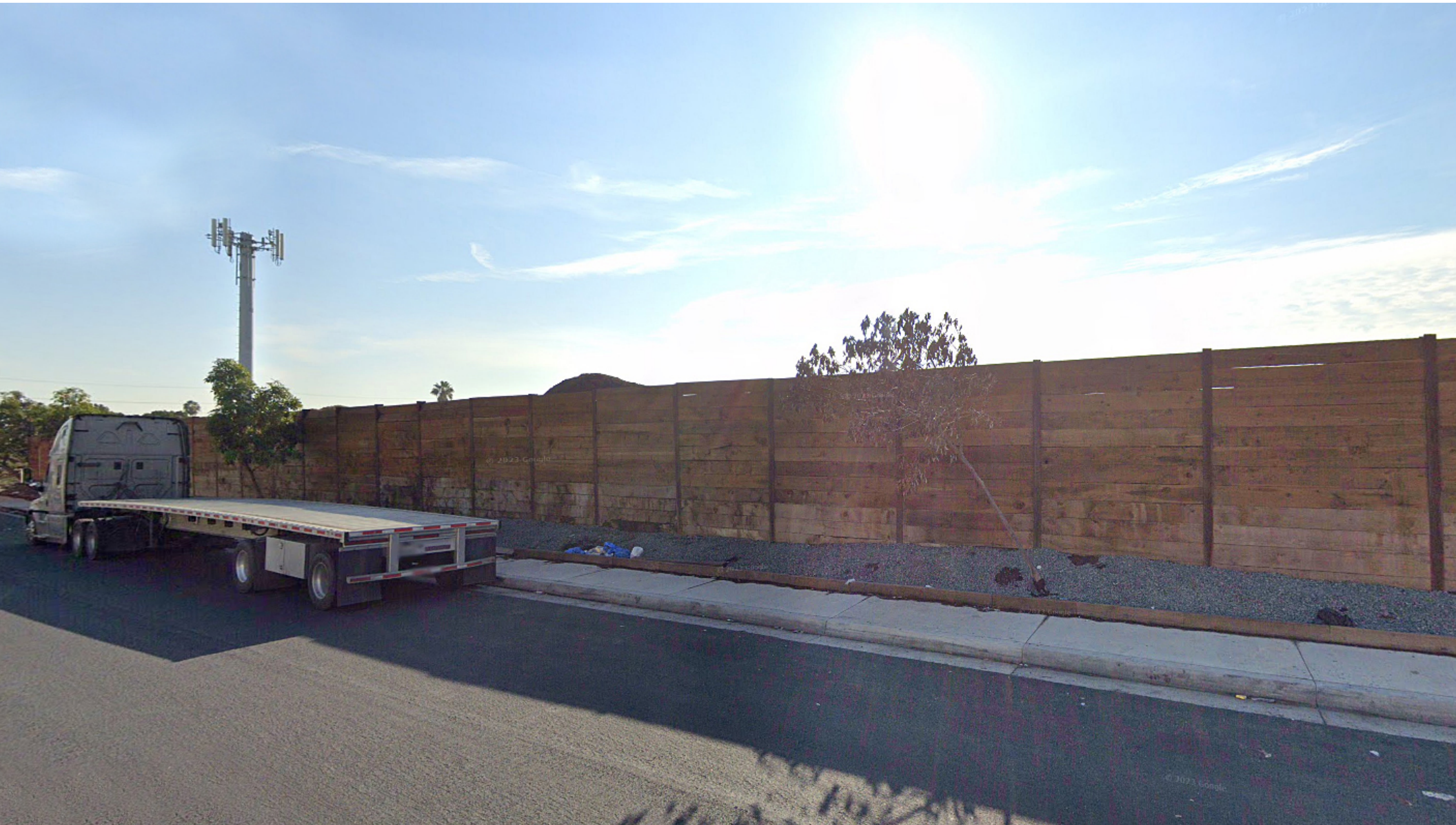
View 2, Existing Conditions Looking SE from West Griffith Street
